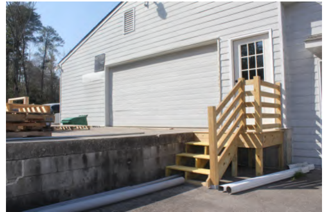
Single and Overhead Door Access
