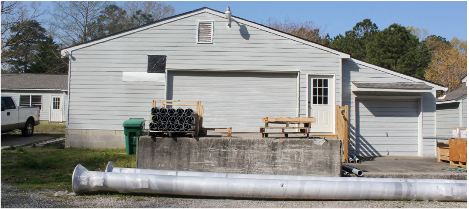
Fronts of 1,660sf Unit (left) and 456sf Unit (right)
