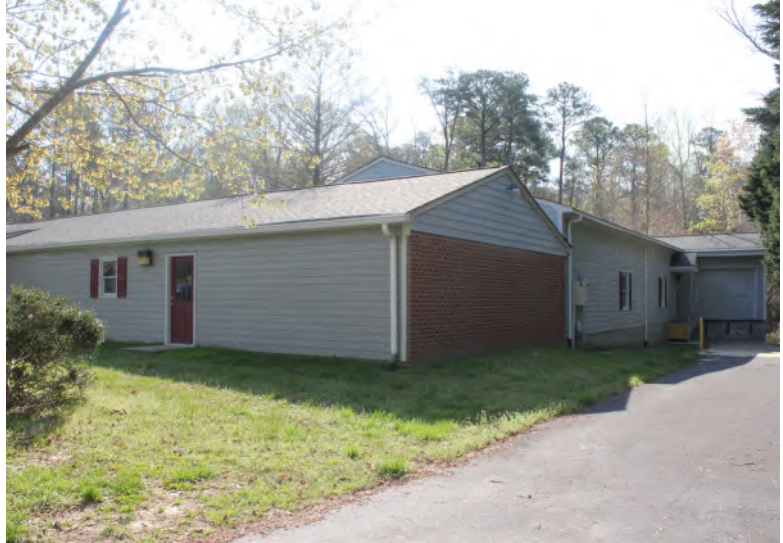
Dock Level Loading Area at rear of space
