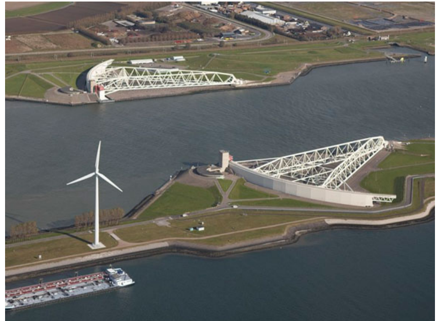
Maeslantkering Storm Surge Barrier, Netherlands Wired Magazine, 2008
